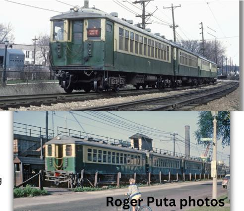
the time, were assigned to all runs through the two subway lines. Being equipped with trolley poles, the cars were also often used on outlying "L" lines and were even leased to connecting electric interurban rail lines. In the 1950s, more modern steel cars were bought, and air conditioning would first arrive on cars ordered in 1964. The wooden cars were all retired, and the 4000s were quickly becoming outdated with the swift advances in technology.
