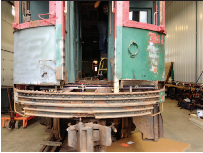
▲ A view of the east end, with the corroded steel cut away in preparation for new replacement steel.
