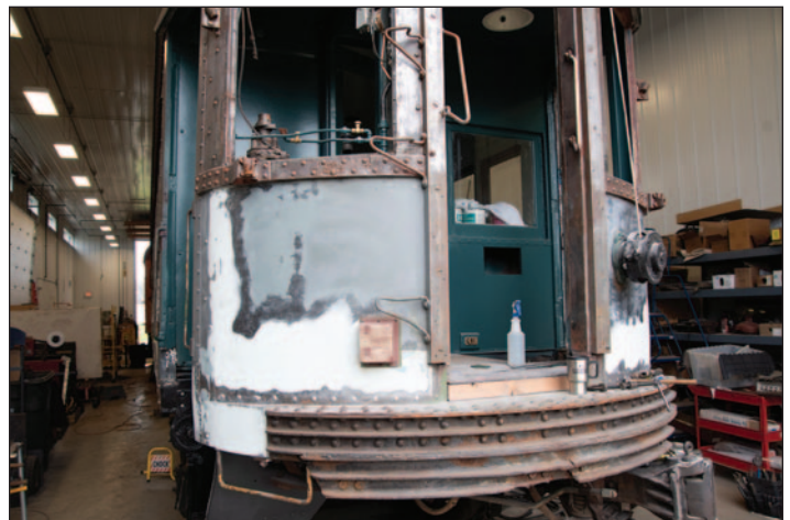
▲ Body filler had been applied over the repaired steel and sanded to prepare the east end for painting.
