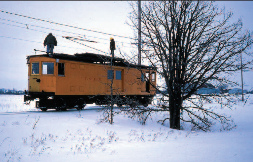
▲ The crew of D-23 makes a repair to the overhead line on January 30, 1982. —Russ Porter photo
