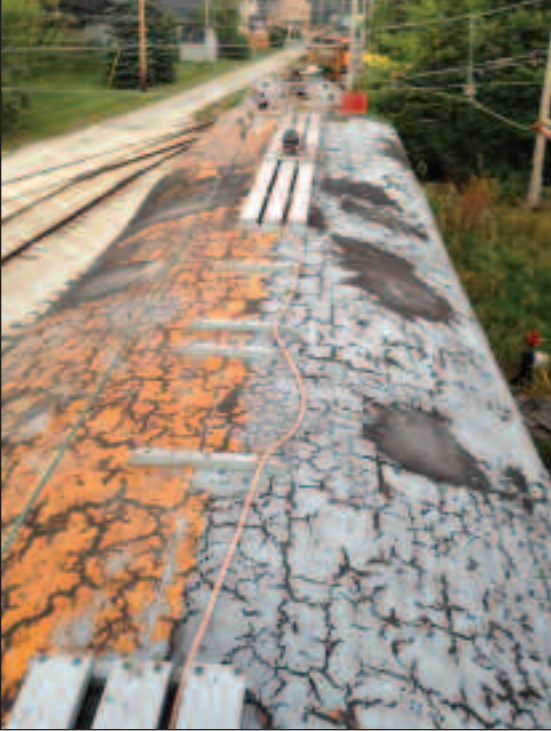
◀ The cracked and multi-colored roof of car 9 in September 2013.
