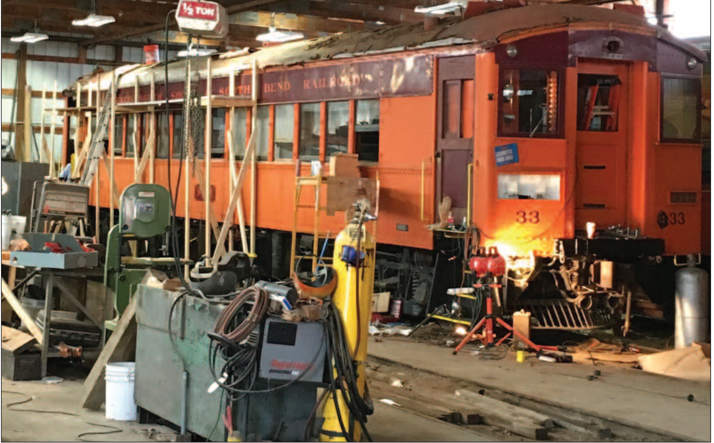
▲ Car 33 is shown in the East Troy car barn, where the restoration took place. The pantograph and most of the vents have been removed from the roof in this photo.
